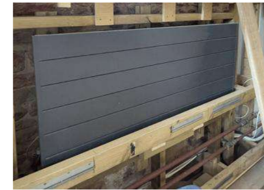
Figure 1: Jaga Briza concealed fan assisted radiator
